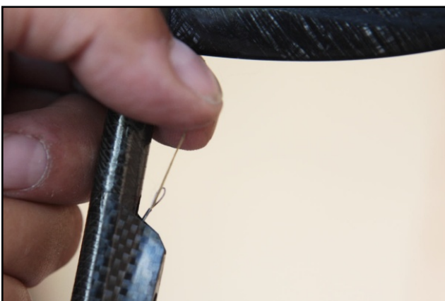
Figure 2.13-The thread on the cable of the elevator
